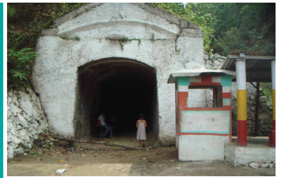
Southern Portal of Churia Tunnel
