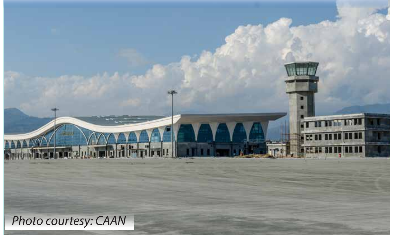
Terminal Building, Pokhara Regional International Airport Project (PRIAP)
